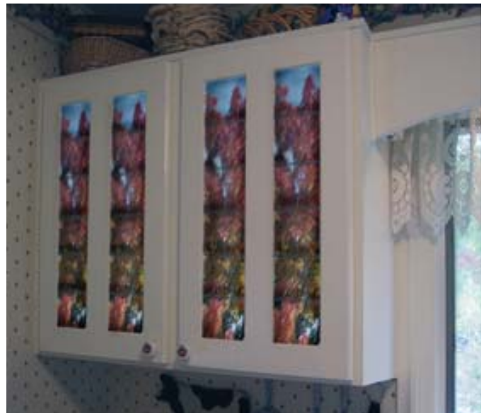
6 x 6 Satin Finish Ceramic Tiles Inlaid on Kitchen Cabinet Doors
